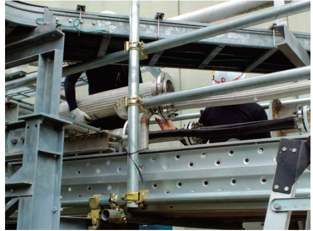
Fig. 4. Exchange work of the He flexible hoses.
