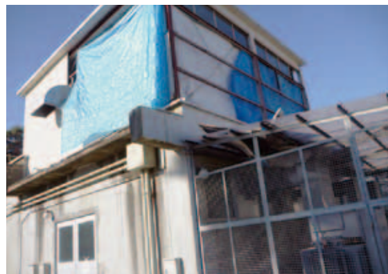
Fig. 6. A wall collapse of the information system center to a power trans retarded recovery of J-PARC information system.
