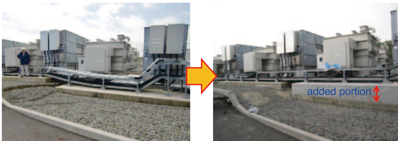
Photo 6. Around the 3 GeV RCS building, a significant amount of concrete had to be added to bring it back to the normal level.
