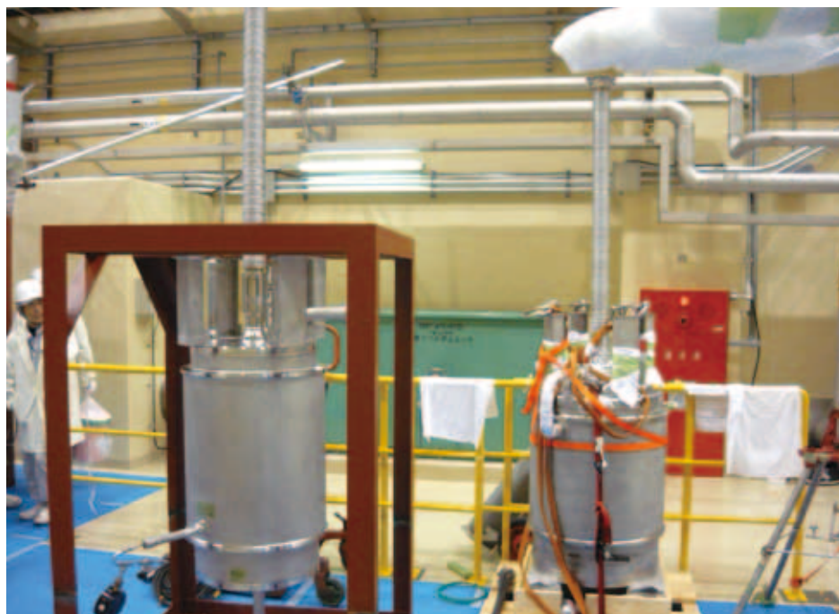
Photo 1. Exchange of the accumulator for cryogenic hydrogen system. The cryogenic hydrogen system was recovered to receive 200-kW beam by exchanging the failed accumulator (right) to new one (left) in the summer shut-down period.
