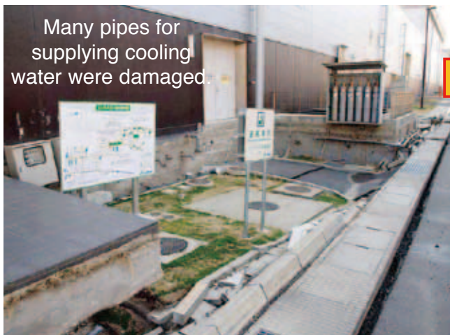
Photo 2. A small place in front of Linac sank by 1.5 m (left). Repair works are under progress (right).
