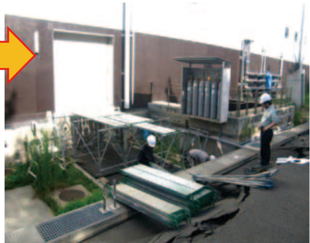
Photo 2. A small place in front of Linac sank by 1.5 m (left). Repair works are under progress (right).
