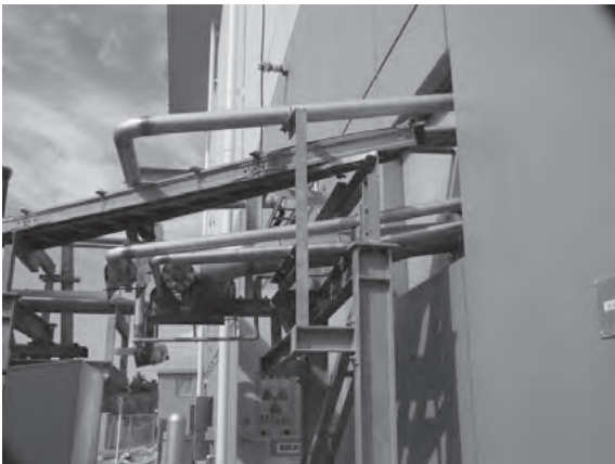
Fig. 11. Damaged helium ducts for the on-line refrigerator at the boundary of the MLF building.
