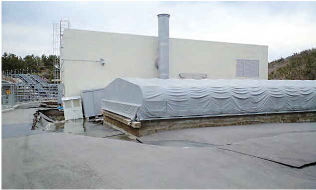
Fig. 1a. The collapsed ground due to the earthquake.
