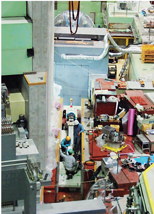
Fig. 1. Realignment of the beamline components of the KOTO experiment.
