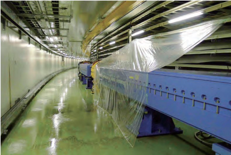
Fig. 4.1. Groundwater leaking in the MR tunnel.
