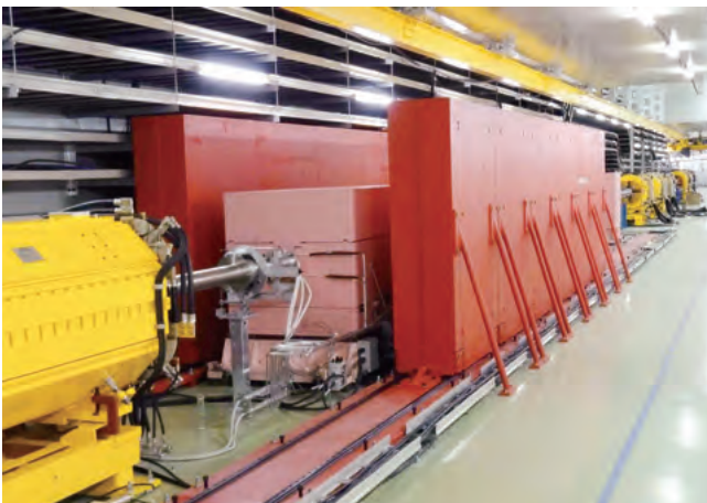
Fig. 4.4. Newly installed iron shields in the MR collimator section.
