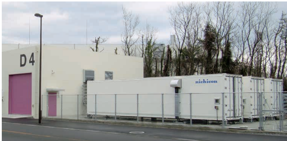
Fig. 17. Capacitor banks at the new building. Three containers contain the capacitors. D4 is one of the new power supply buildings.
