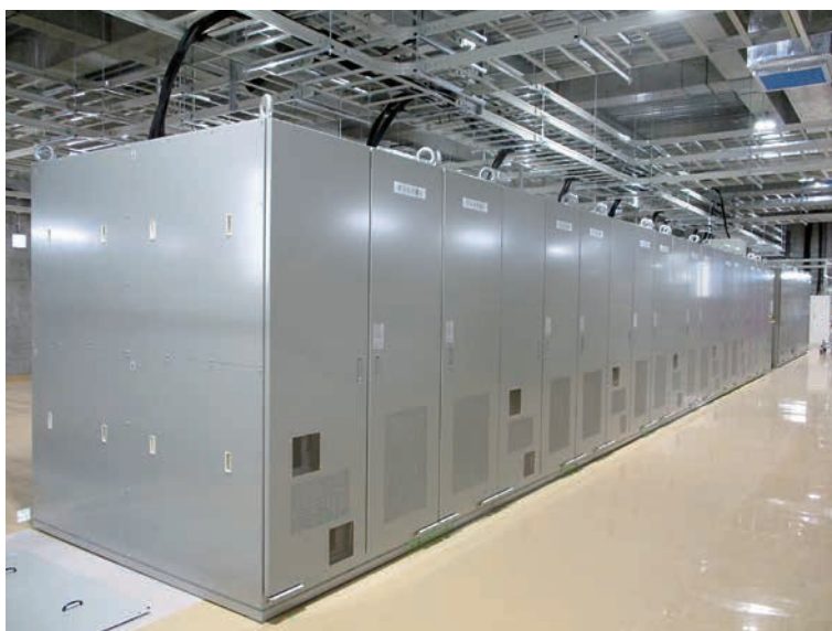
Fig. 16. New power supply for the bending magnet Size: W 2.5 m x H 2.5 m x L 25 m
