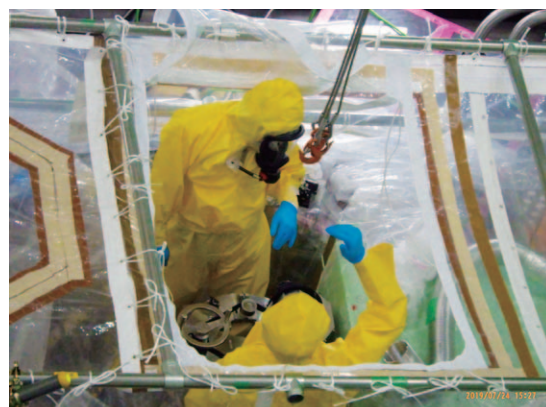
Fig. 2. A snapshot of the MUSE target team working on the target replacement assembly, where the radiation workers wearing airtight suites are in a temporary greenhouse to contain radioactive contaminants.
