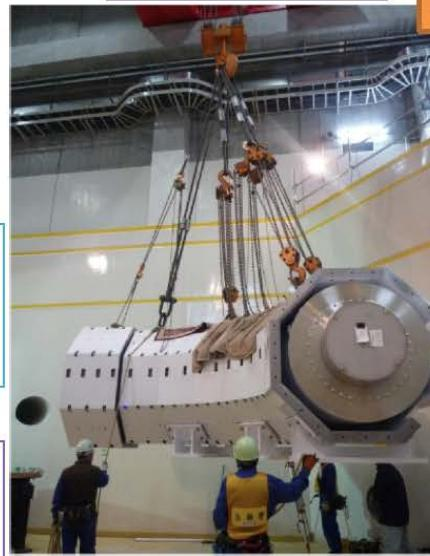
90 deg. Transport Solenoid installed in Spring 2015
