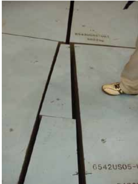
Displacement of shielding wall in MLF. The 2 nd Hall: BL20 Area (upper) The 1 st Hall: BL04 Area (left)
