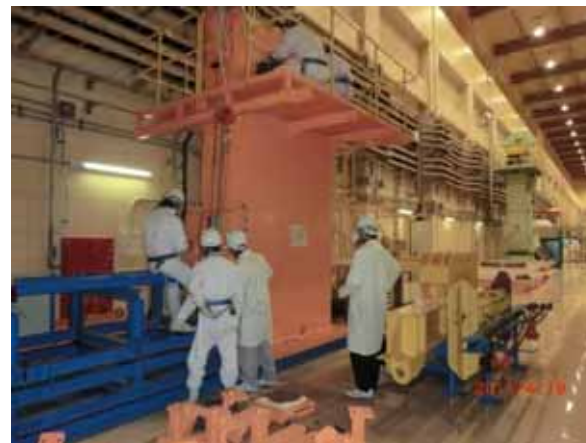
Inspection of Shutter blocks with crane.
