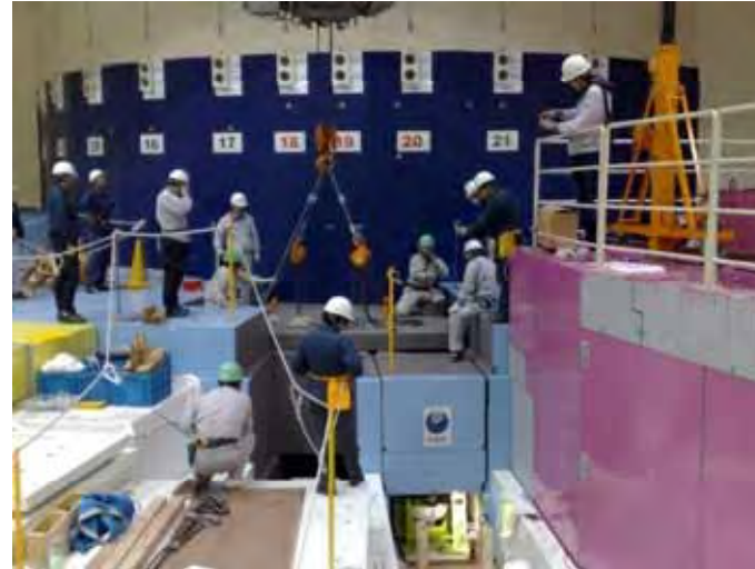
Operation of how removal was done.
