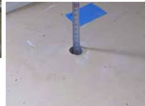
One room on the side. By digging a hole, 50 cm hole (gap) was detected.
