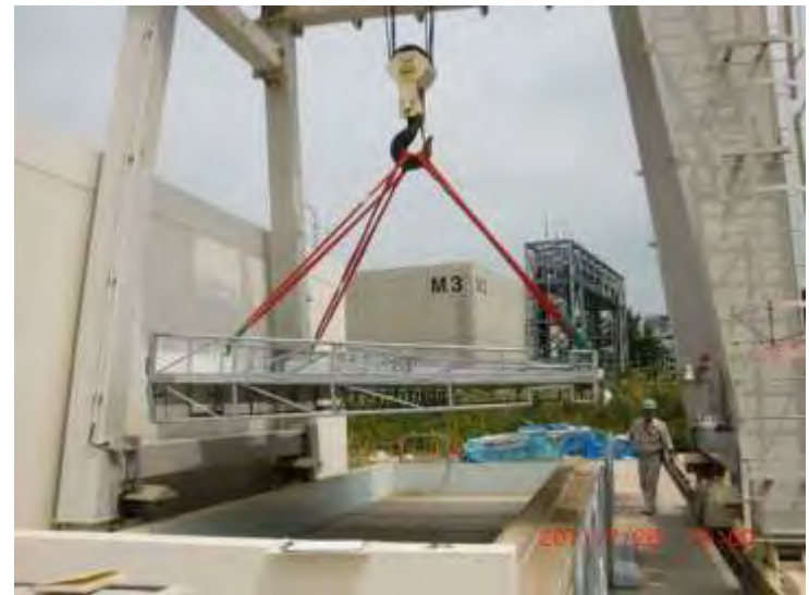
Crane at Bring-In Entrance
