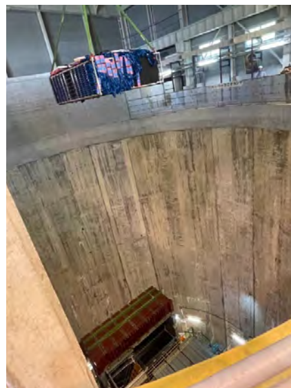
Fig. 1. Installation of SuperFGD into the near detector.
