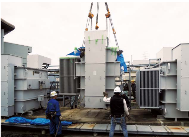
Fig. 12. Installation of the new transformer-rectifier
