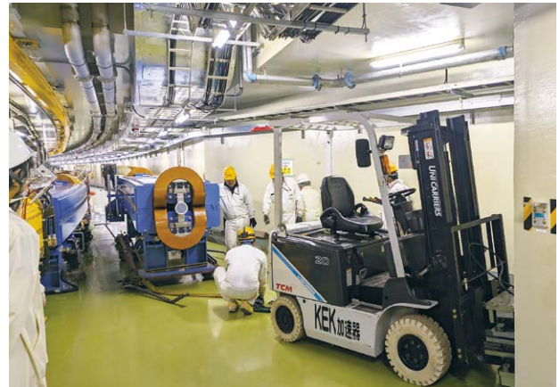
Fig. 17. Replacement work of the main bending magnet
