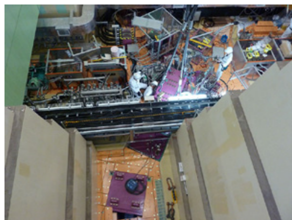
Fig. 21. A picture of the installation of the HS1, HS2, HS3 and HB1 in the vicinity of the muon target.
