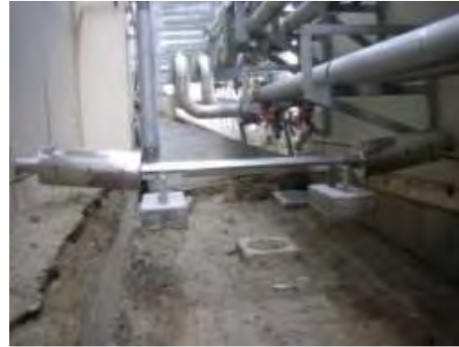
↑ Disconnected pipes Distortion of bellows →
