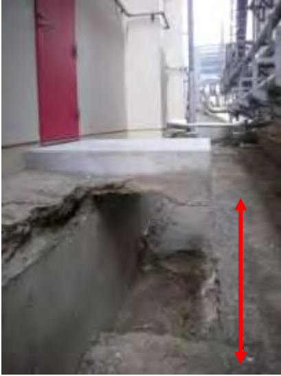
← Entrance for the Hall. About 1 m gap.
