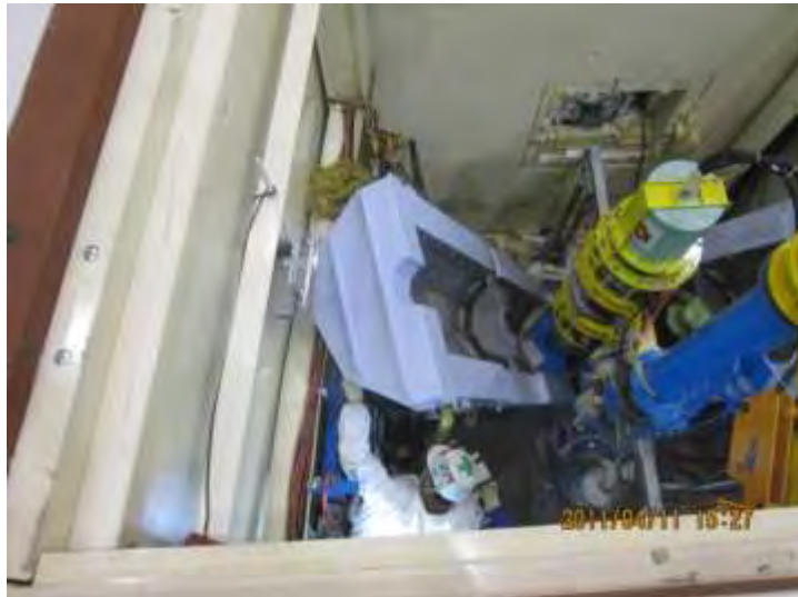
↑ Removal of Pb shield wall.
