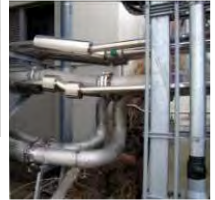
↑ Disconnected pipes Distortion of bellows →
