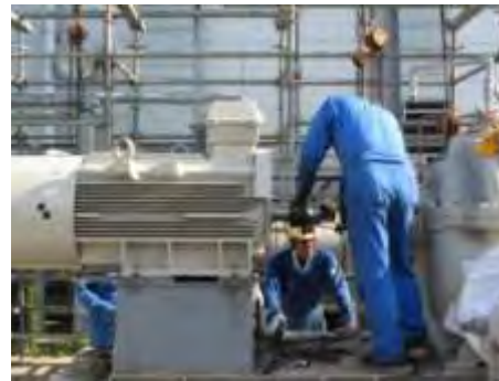
Reinforced foundation for a cooling tower (right) Adjusting alignment of pump/motor (left)
