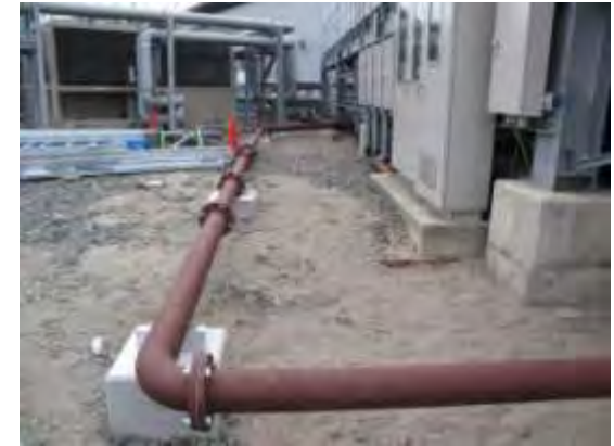
Damaged water pipes were replaced to enable cooling.
