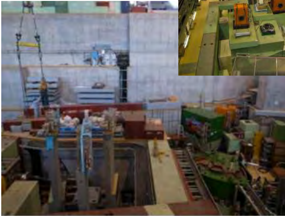
Inspection work in Hadron Hall
