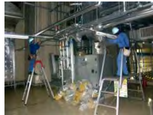
Restoration work on power supply
