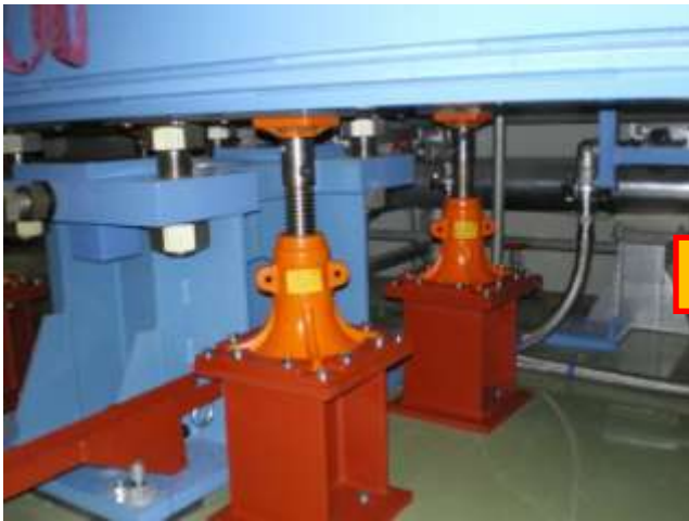
Jacking up an electromagnet to make a space between the magnet and the stage
