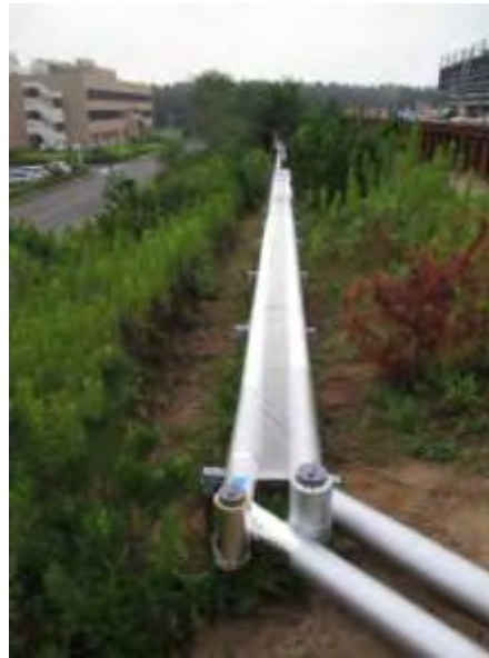
Damaged water pipes were replaced to enable cooling.
