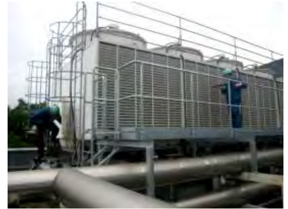
Cleaning work on cooling water tanks
