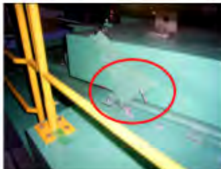
BL15 Damage of upper shielding clasp
