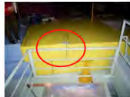
BL18 Shearing and falling of shieldings
